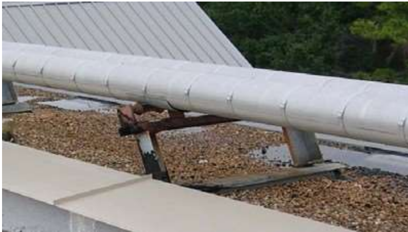
Inadequate design to manage thermal expansion & contraction
