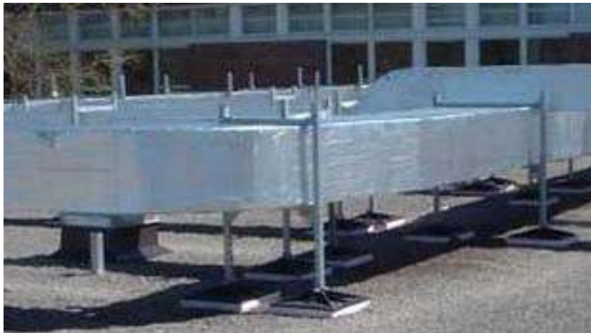
Enclosed duct supports
