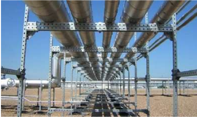
Open pipe support system with straight bracing
