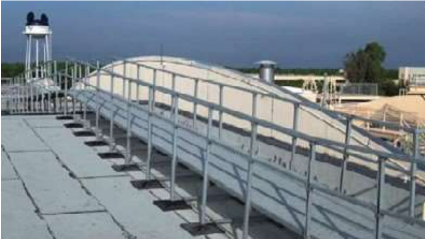
Walkway system, 4' wide, raised 30" off roof
