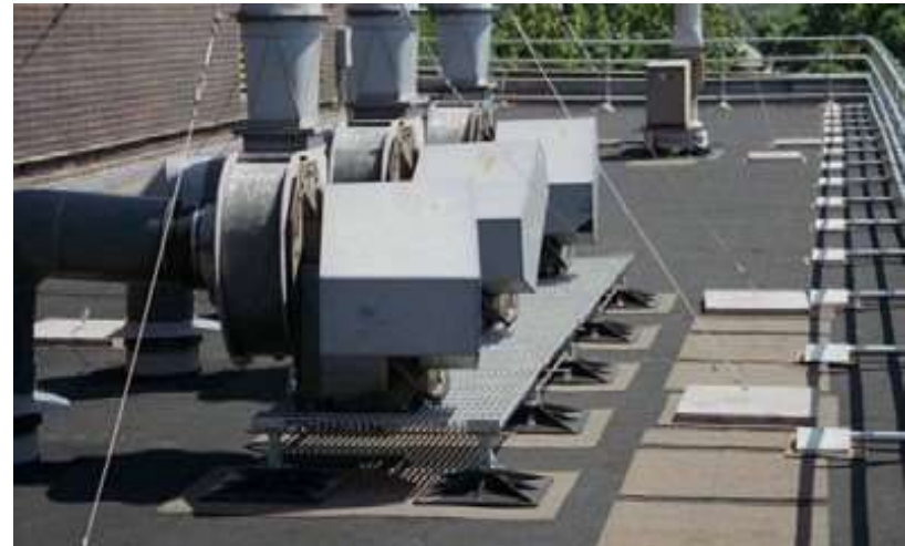
Equipment platform supports for blowers
