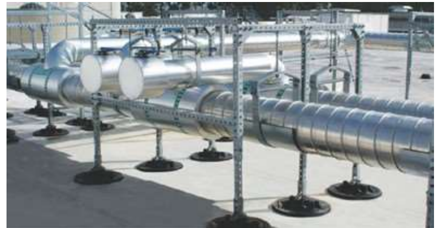
Multiple hanging gas piping with center leg support
