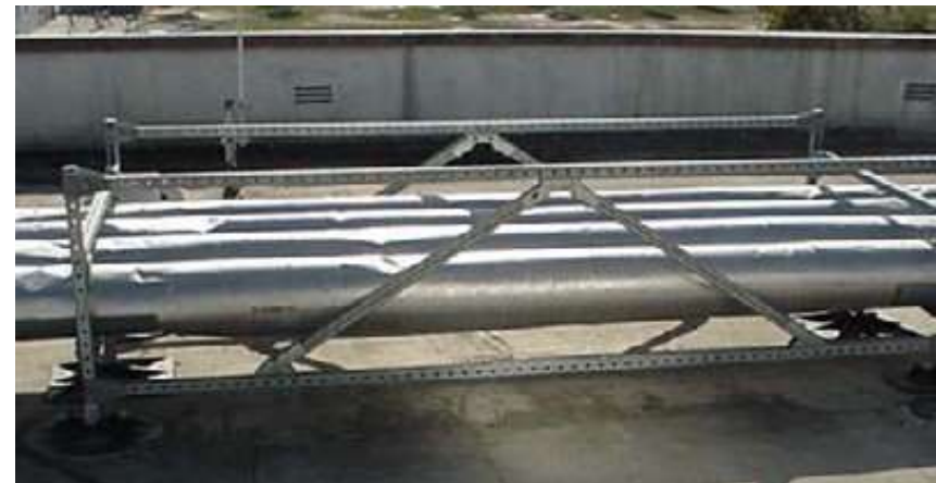
Enclosed pipe support system with k-bracing
