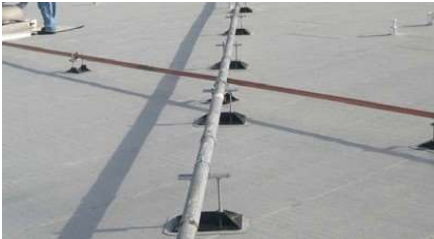
Height adjustable supports (adjustable to 10")
