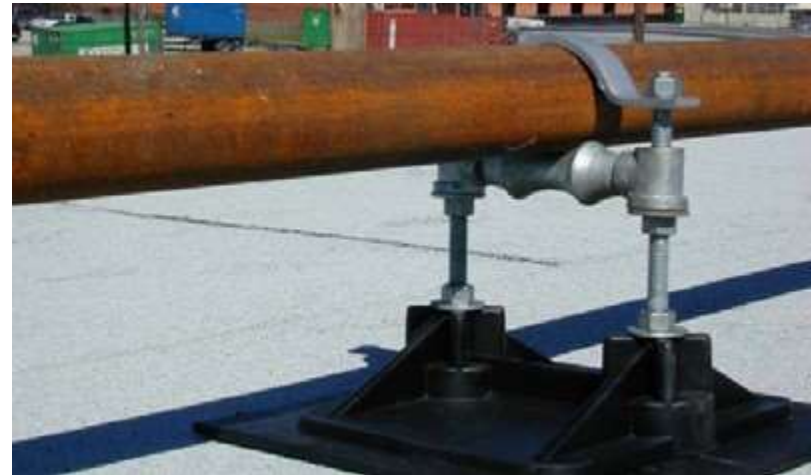
Height adjustable supports with roller and pipe guide
