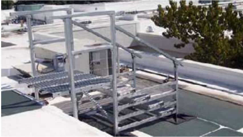
Roof-to-roof access stairs with handrails
