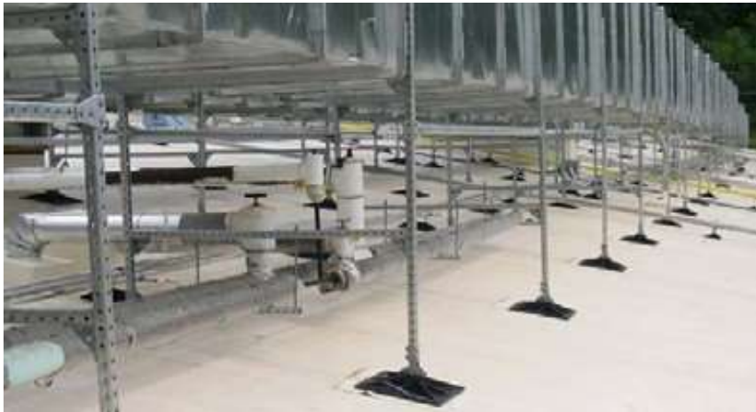
Open duct supports with swivel assembly, adjustable supports and pipe guides on sloped roof
