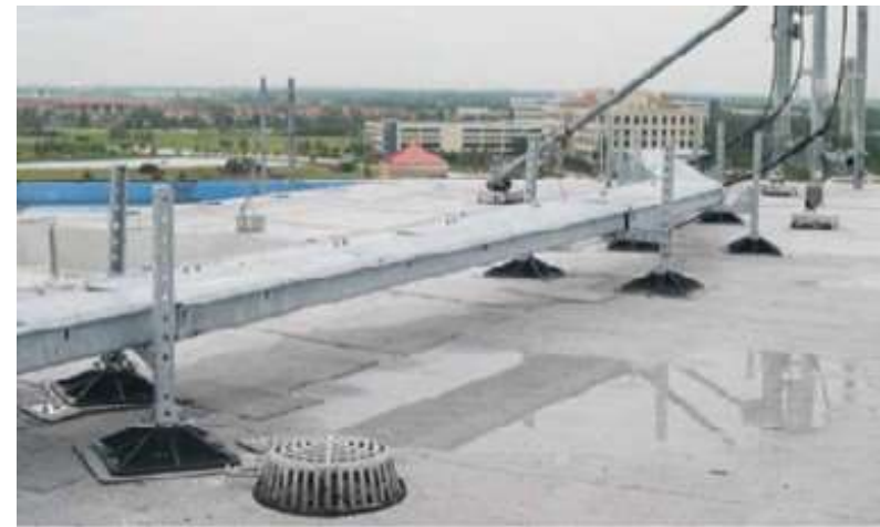
Cable tray raised 12" off roof
