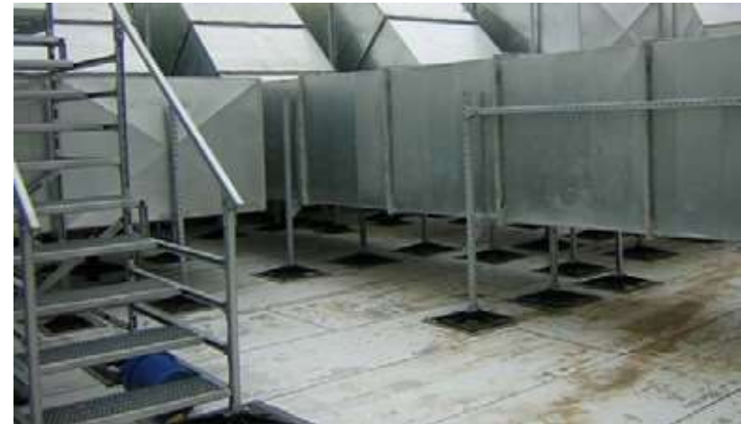
Open duct supports with straight bracing and crossover system
