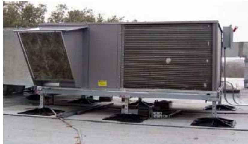
Multiple 10 and 15-ton rooftop units with center and corner equipment supports raised 10" above roof
