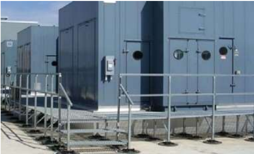
Access platform with stairs
