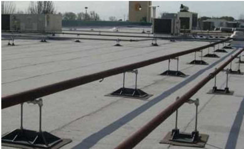
Height adjustable supports with rollers
