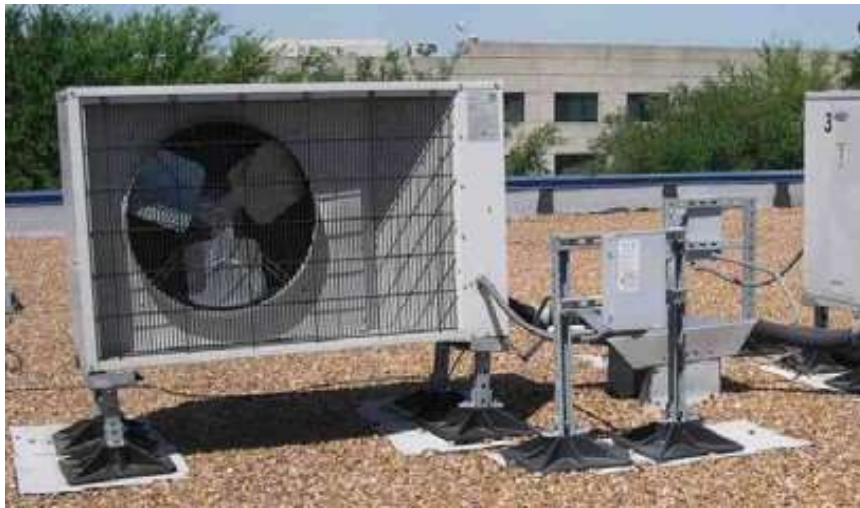
Rooftop blowers with corner supports and AC disconnect supports
