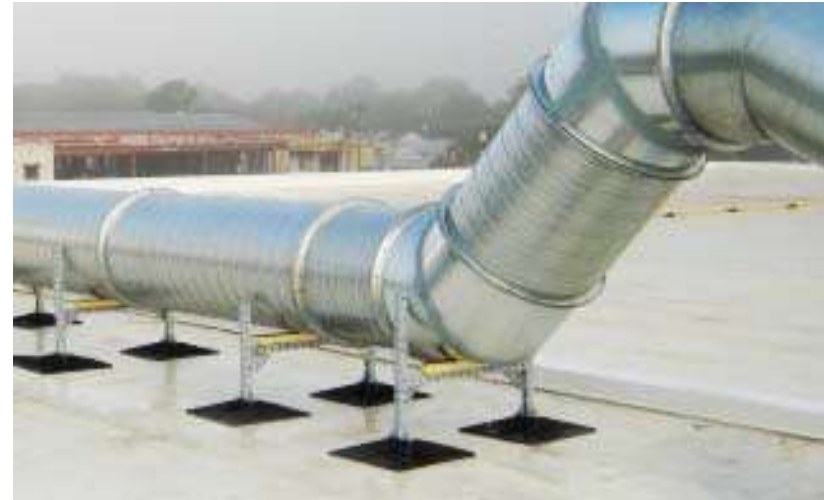
Open duct supports
