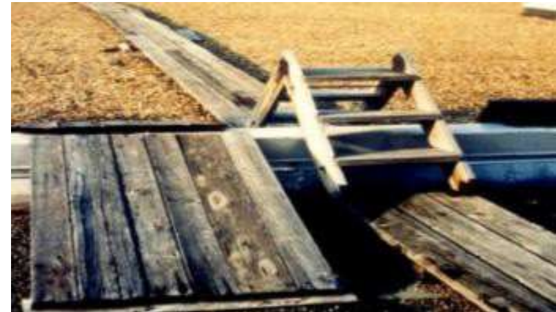
Inadequate walkway causing roof penetrations
