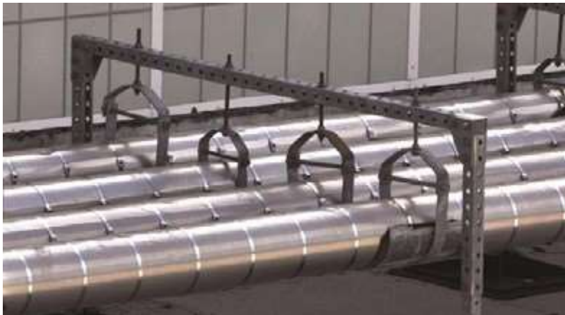
Multiple hanging gas piping
