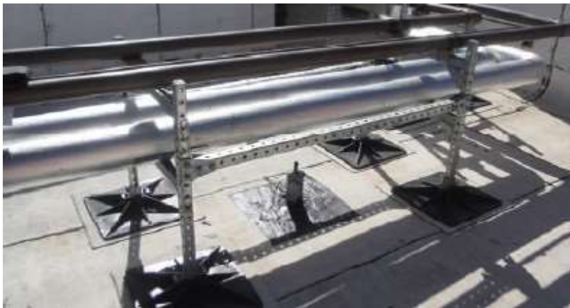
Open & Enclosed pipe support system with straight bracing
