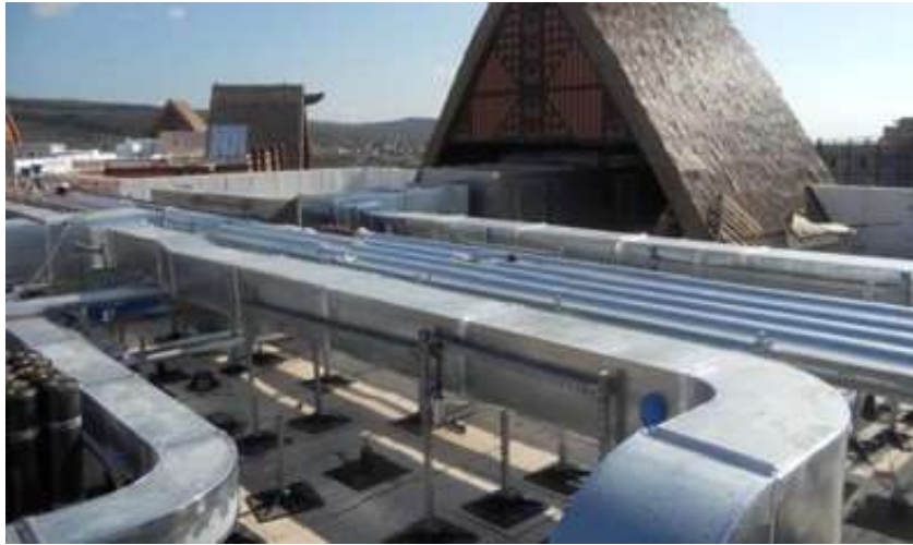
Duct and pipe support system with straight bracing
