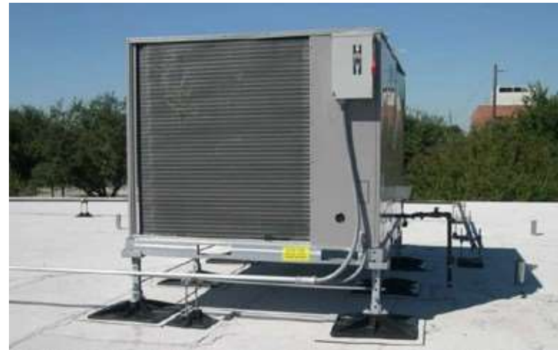
HVAC with corner and center supports and with electrical and gas supports
