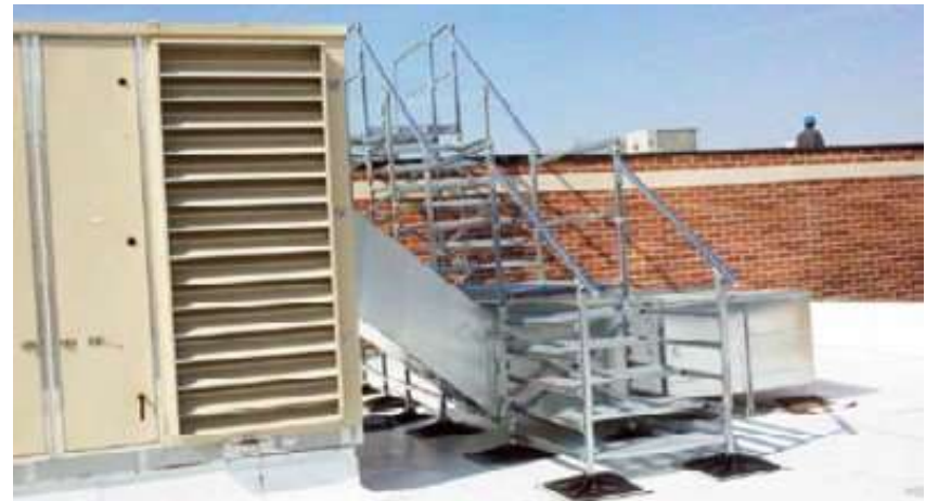
Crossover, spanning duct supports and 6' retaining wall
