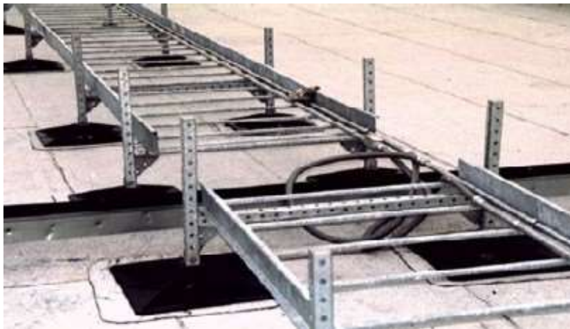
48" wide cable tray at 12" off roof
