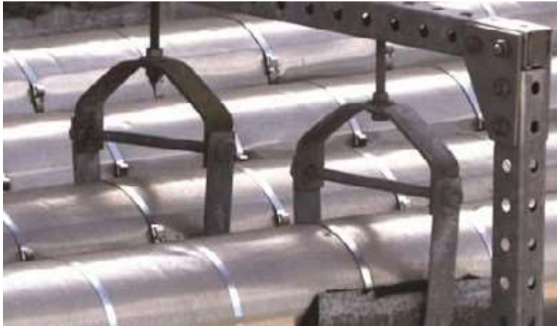
Pipe supports with clevis hangers
