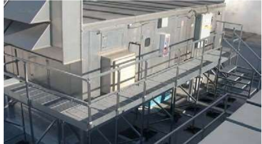
Walkway system with OSHA railing and stairs
