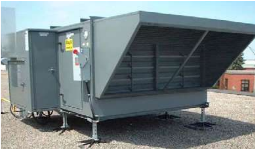
10 and 15-ton rooftop units with corner equipment supports raised 10" above roof
