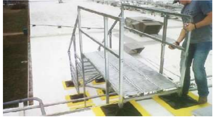
Roof-to-roof access stairs with handrails
