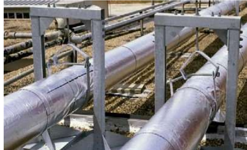
Inadequate design to manage weight
