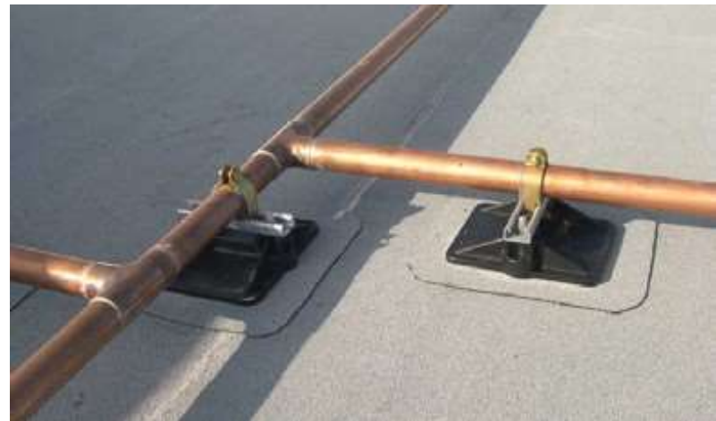
Non-adjustable support with channel
