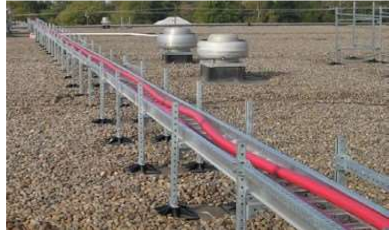
Over 3,000 lineal feet of cable tray ranging from 12" to 36" wide and 36" above finished roof
