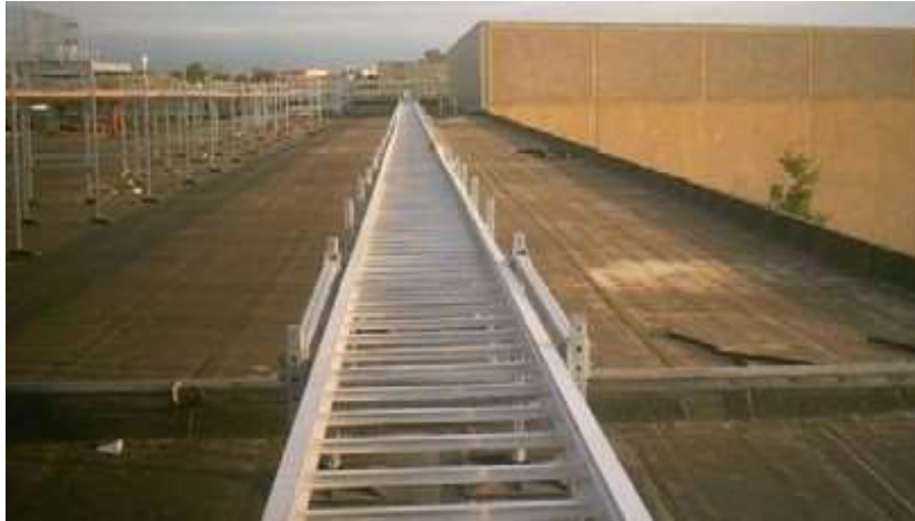
Over 3,000 lineal feet of cable tray ranging from 12" to 36" wide and 36" above finished roof
