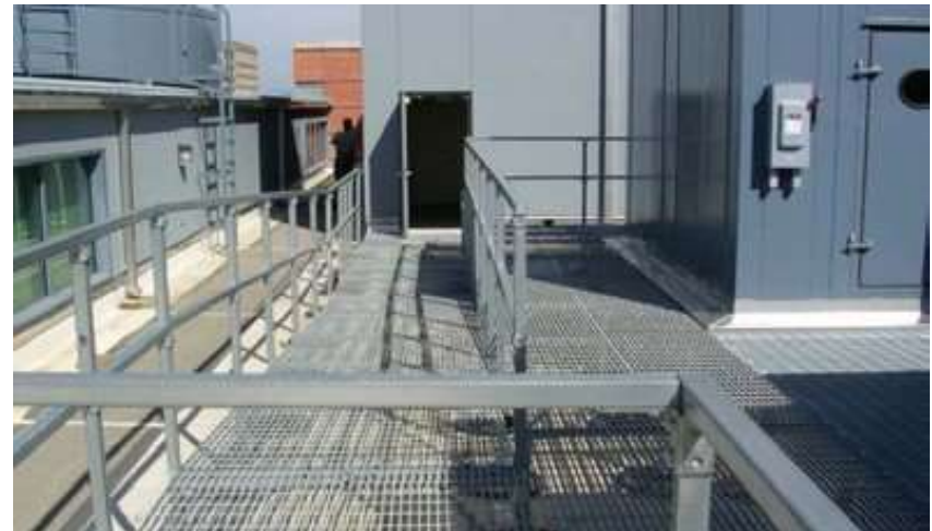
Ramp and walkway system with handrails
