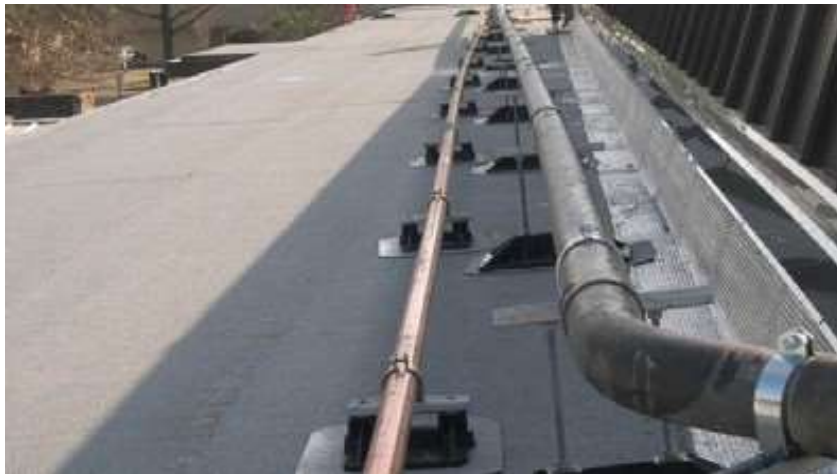
Non-adjustable supports with channel and pipe guides
