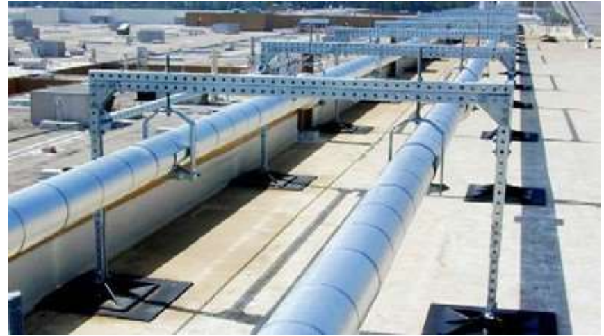
Multiple hanging gas piping
