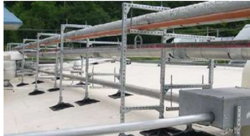
Enclosed pipe supports and custom hanging supports with clevis hanger and swivel assembly
